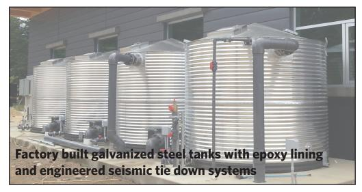
**Gabriola:** 4 - 3750 US gallon galvanized steel epoxy lined tanks for toilets, vehicle wash, and emergency water supply.
