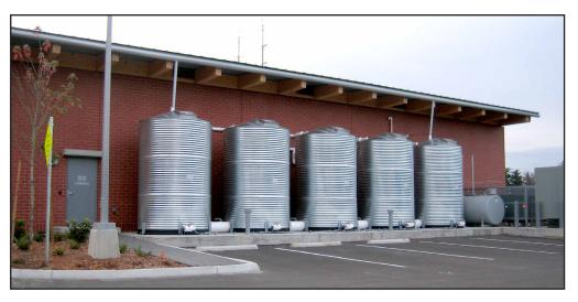
**Central Saanich:** 5 - 3718 US gallon galvanized steel epoxy lined tanks for toilets, vehicle wash, tanker fill, and emergency supply.
